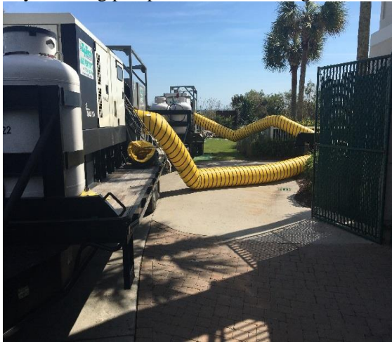
Dry air being pumped into the buildings to remove moisture:
